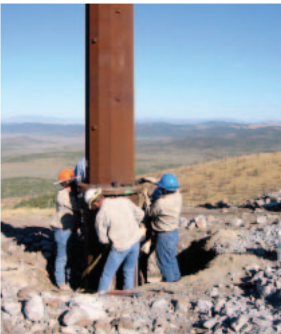
Falcon Gondor foundation installation.
